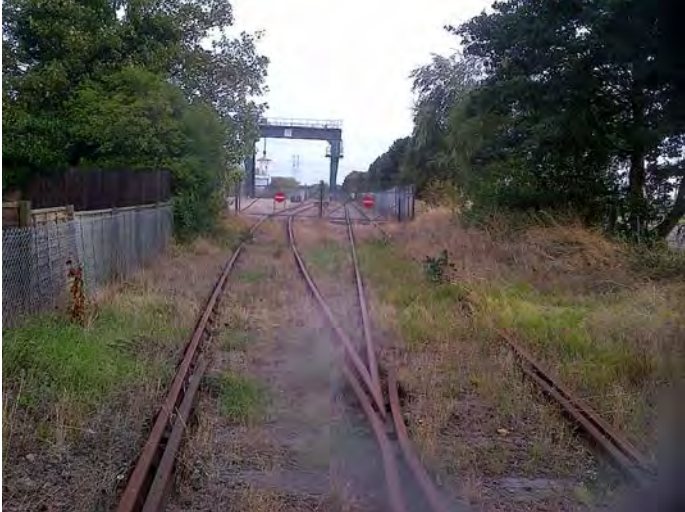
D33 – Photo showing gates at NR Boundary (95M 1634y)
