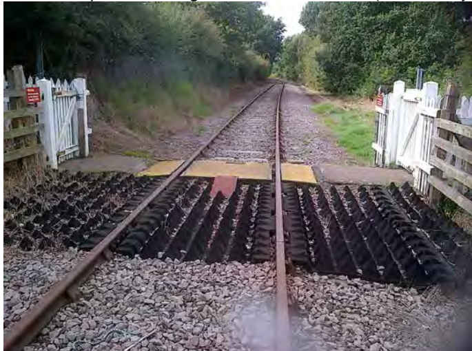
D17 - Footpath crossing 5272.7m – 5273.9m (94M 1445y – 94M 1447y)
