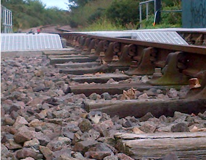
D28A - Longitudinal timber bridge 6249m 6260.2m (95M 748y – 95M 761y)
