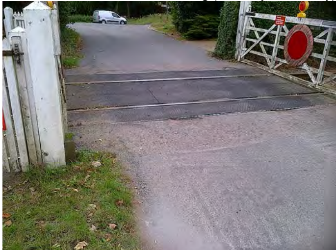
D16 - Saxmundham Road Crossing (94M 39y – 94M 46y)
