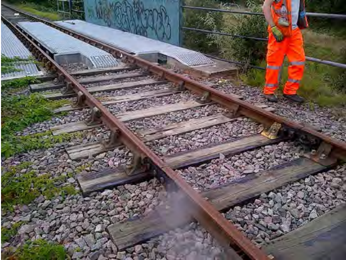
D28D - Longitudinal timber bridge 6249m 6260.2m (95M 748y – 95M 761y)
