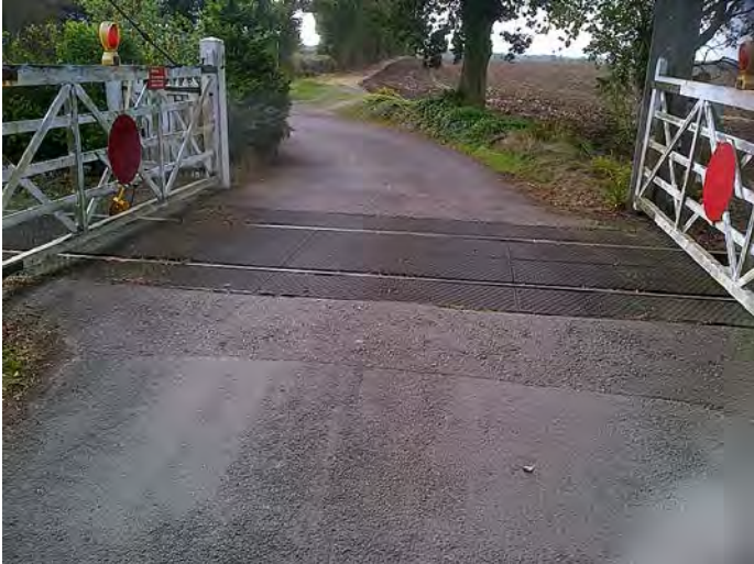
D8 - Knodishall Crossing (92M 1075y – 92M 1083y)
